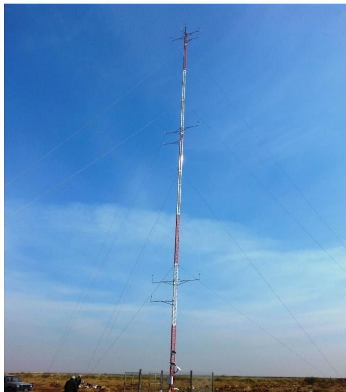
Fig (2) Towers of the Science and Technology Ministry in Al-Shihabi
